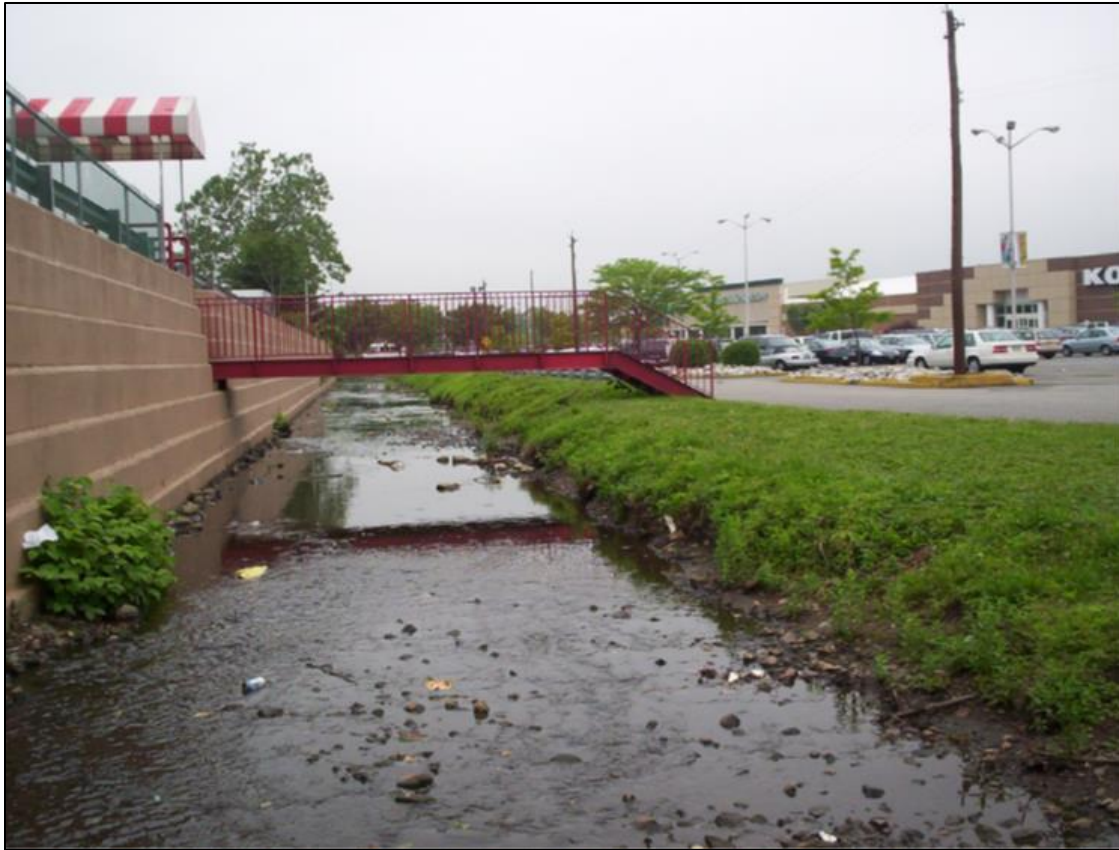
Photo 12: Downstream View of Great Notch Brook within Shopping Center Parking Lot
