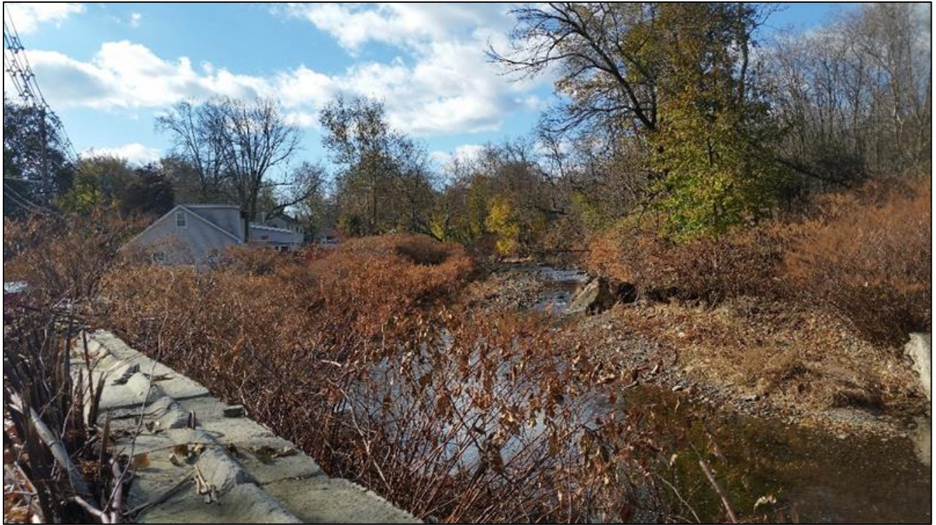
Photo 5: Upstream View of Peckman Along Cedar Grove Rd Near Camp Bal Pl.
